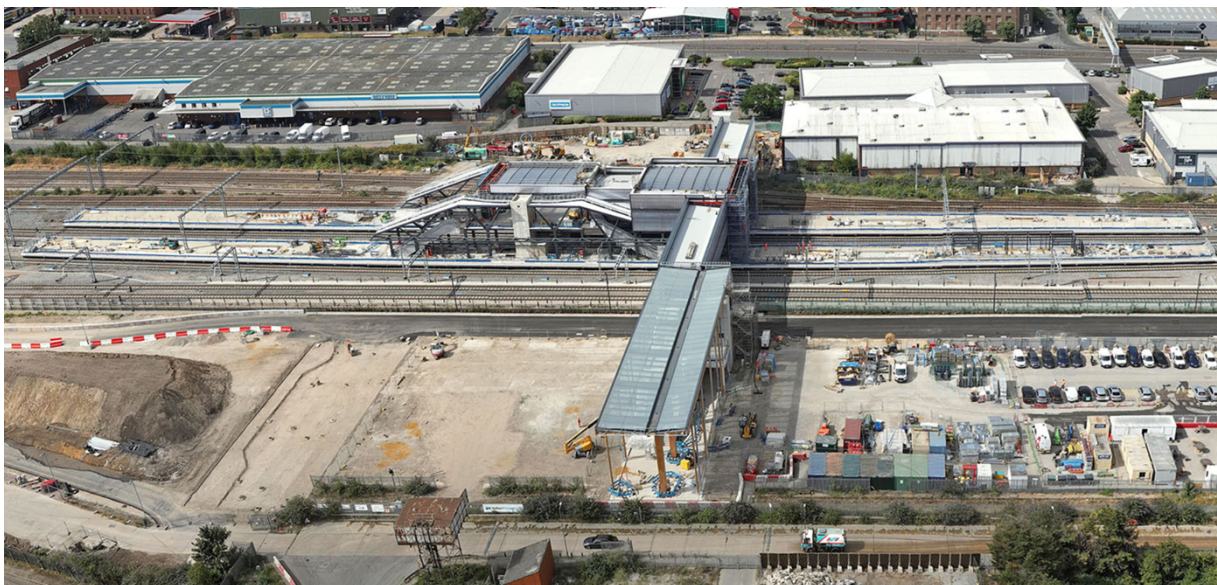
Figure 1 - Brent Cross West Station (July 2022)
